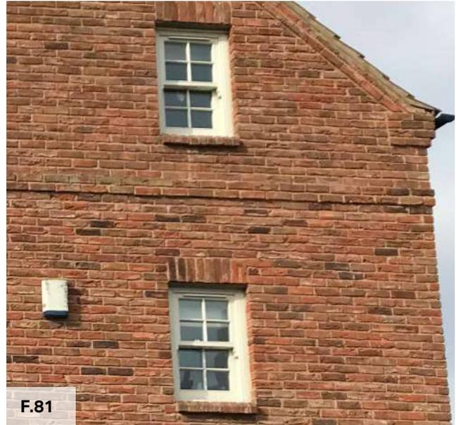
**Figure 81:** Sashes with glazing bars on a red brick house on North Green
