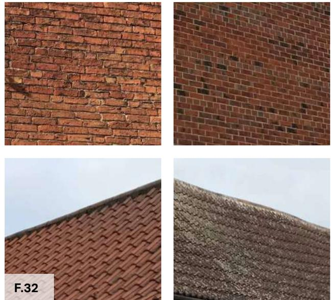
Figure 32: Traditional red brick (top-left), modern red brick (top-right), red pantile (bottom-left), concrete tiles (bottom-right)
