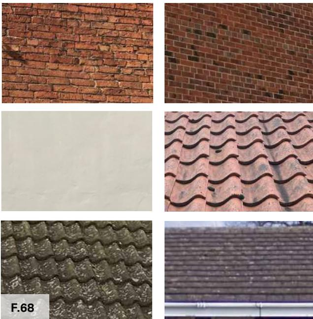
Figure 68: Traditional red brick (top-left), modern red brick (top-right), render (centre-left), red pantiles (centre-right), concrete tiles (bottom-left), slate tiles (bottom-right)
