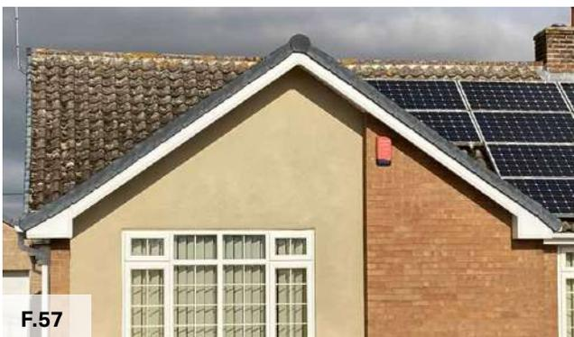
Figure 57: Concrete tiles roof with UPVC roof fascia
